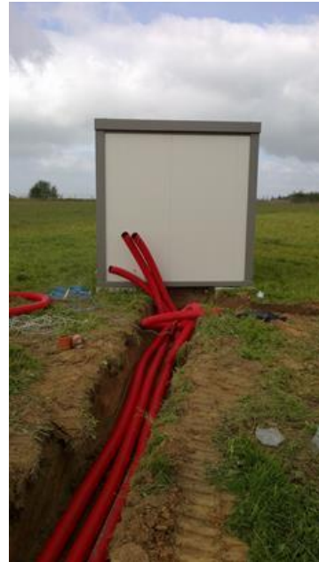
Figure 43: new container installed in Humain and trenches to install the new low-loss cables.
